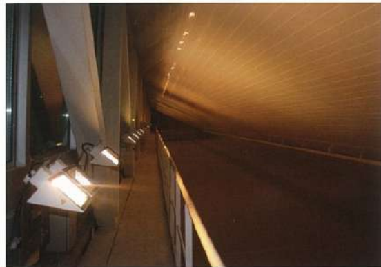
Plano inclinado reflector, tela difusora e estore invertido Slanted reflecting panels, diffusing canvas and inverted blinds
